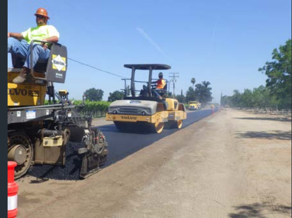
Road Rehabilitation of Road 100 (Akers St.)
