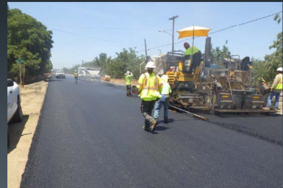
Road Rehabilitation of Ave 256
